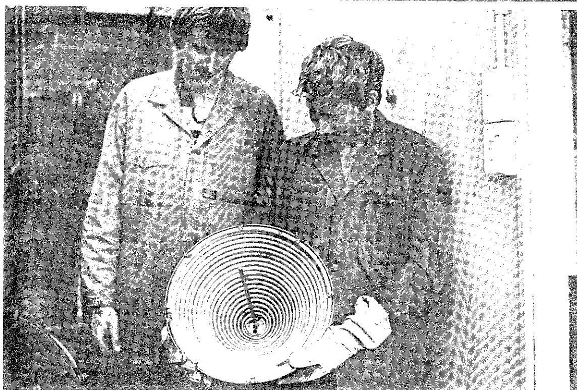
Figure 59(a) Winding a Mark III absorber
