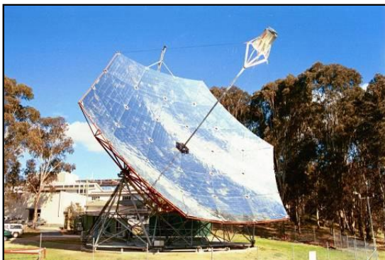
Fig. 1. The existing SG3 400m 2 dish (left) and a CAD image of the new 500m 2 SG4 dish at approximately the same scale.
