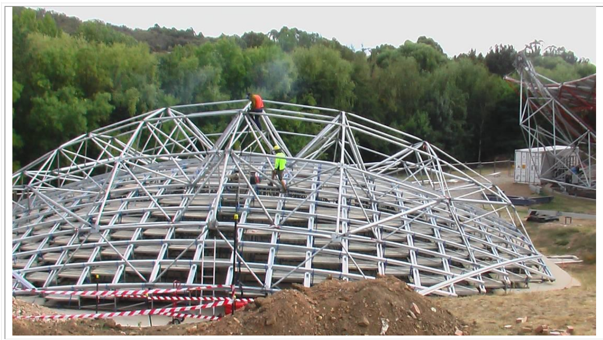
Fig. 4. Dish frame with pyramids installed and back surface chords being welded in place.
