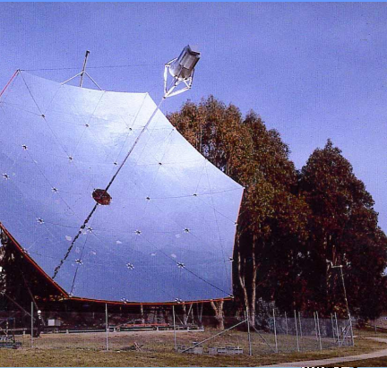
Array of ANU's 400m 2 Paraboloidal Solar Collectors
