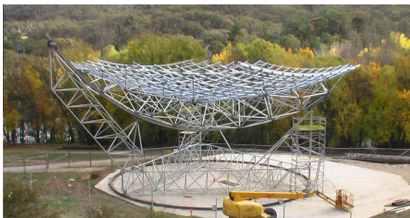
Fig. 4. Dish frame assembled on base-frame, with actuation systems in place.
