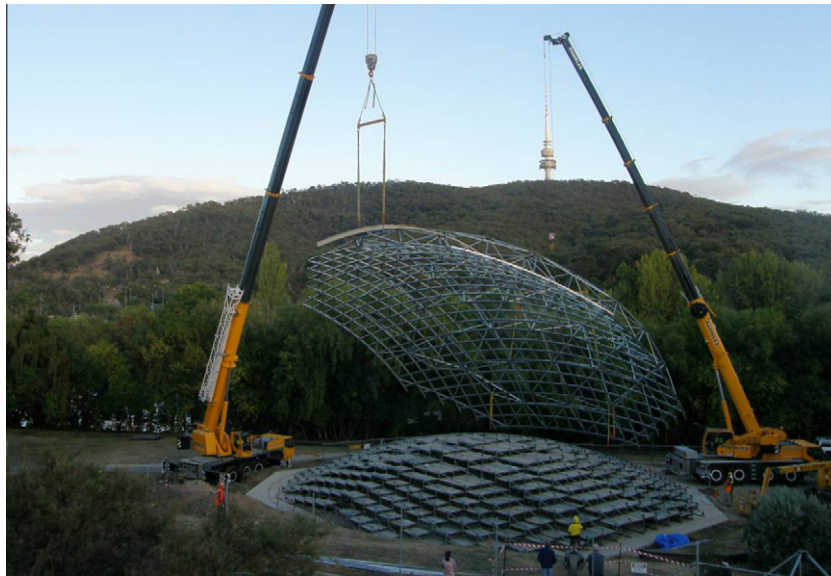
Fig. 3. Removal of the completed dish frame from the jig.
